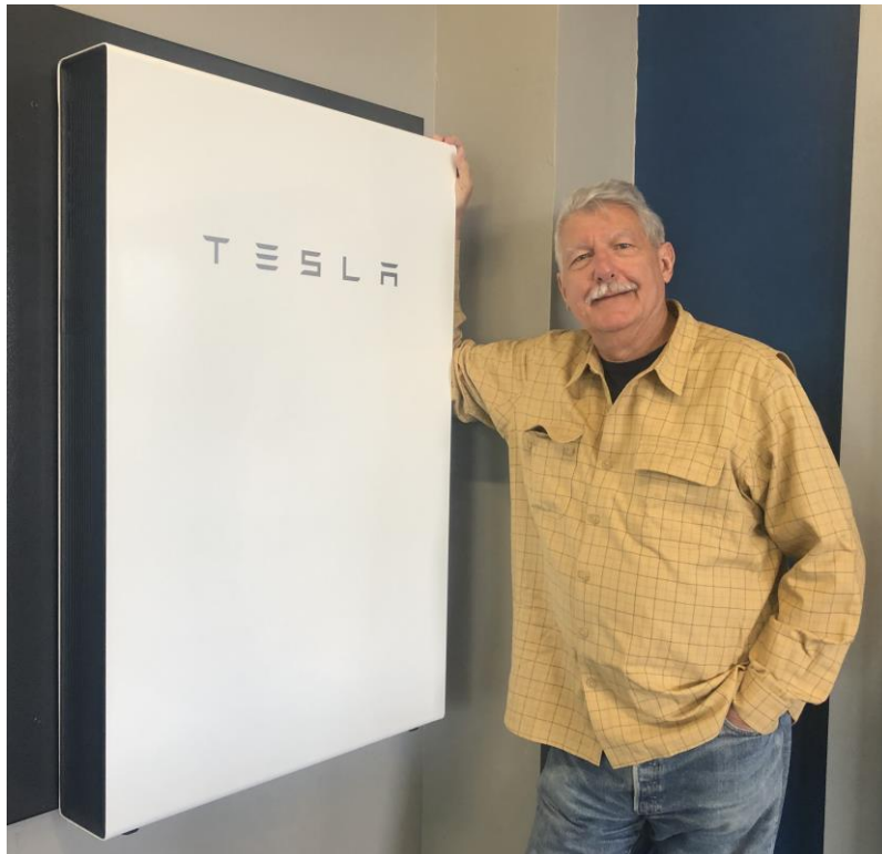
13.5 kWh Powerwall, Enough Juice to Run My House for a Day and I have Six of These
